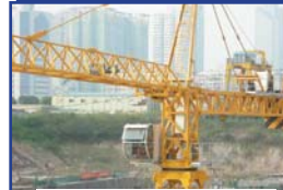
Tower Crane (R7500)
