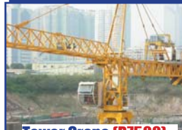
Tower Crane (R7500)
