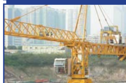
Tower Crane (R7500)
