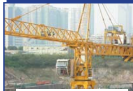
Tower Crane (R7500)
