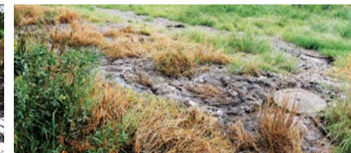
Another manhole where more solid sediment had recently spewed from.
