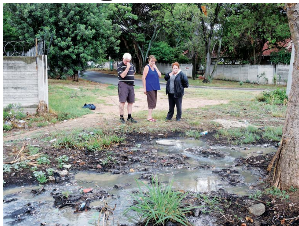
A rotten foul smell seeps out of another blocked sewage pipe in Geelhoutpark; these blockages have become a familiar scene to locals. On the photo from left; Jon Gowland, Suzie Gouveia, and Sharon Gowland.
