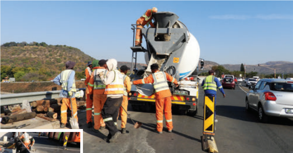
Temporary lane closures allow cement trucks and construction vehicles safe access as work continues on the Helen Joseph Bridge project.
